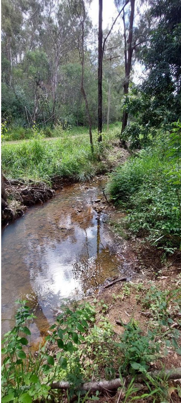
Accumulated bed sediment in reach above bridge, a target for extraction and channel capacity reinstatement . Road frontage in background currently experiences flooding when the stream breaks our of the sediment filled channel.
