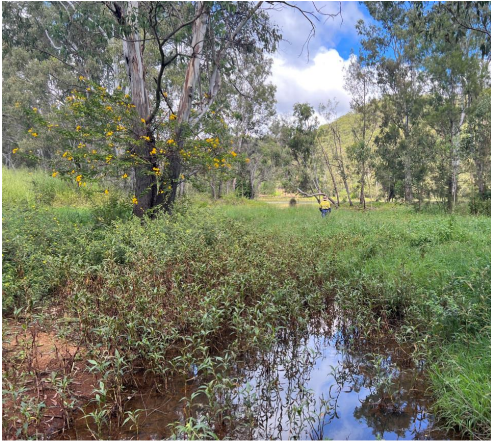
Figure 24 Sediment accumulation and colonisation in the sediment forebay of the Loudoun Dam
