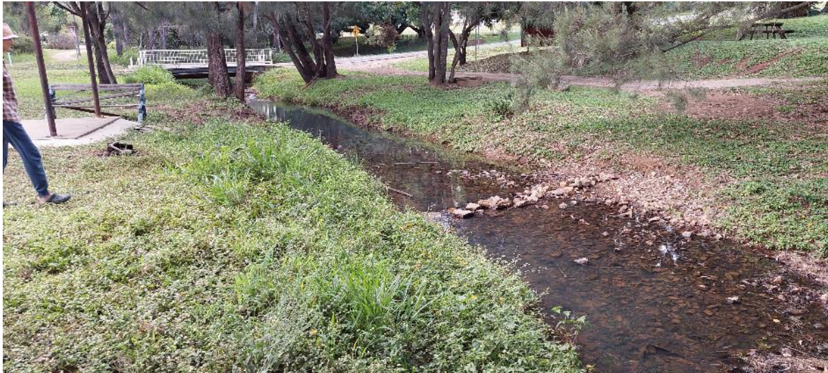
Proposed swimming pool feature would lie to left in front of upstream bridge crossing. Protection and stabilisation of bridge infrastructure under high flow events needs to inform pool design.
