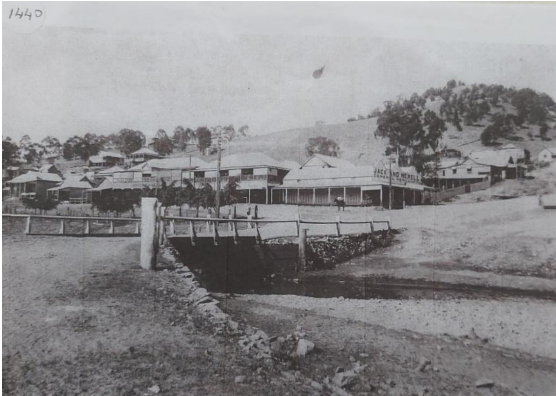
Figure 2 McDonald Creek Bridge Crossing in 1914, from downstream looking upstream
