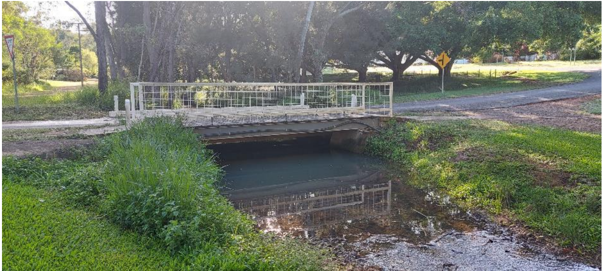
Constricted scour pool beneath existing MacDonalds Ck bridge – currently used for swimming recreation. Emulation of flow constriction – scouring pool formation proposed for upstream reach
