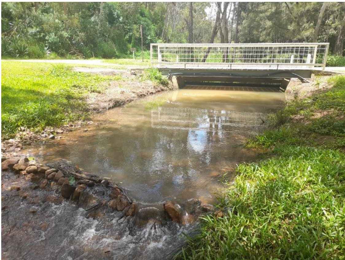
Figure 1 McDonald Creek Bridge Crossing in 2021, from downstream looking upstream
